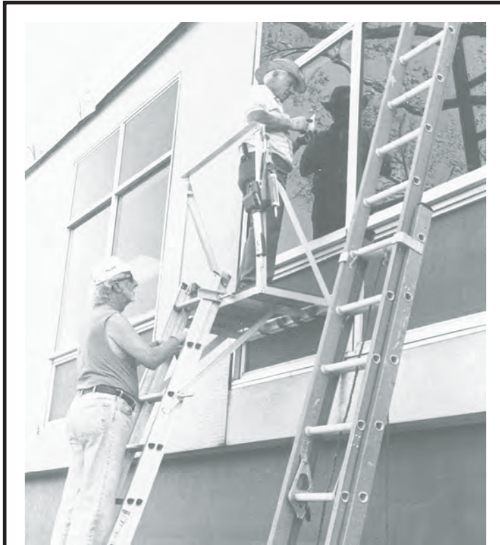
SPRING MAINTENANCE —Workmen calk new windows at the Diocesan Patoral Center, Boise. The windows are part of a general maintenance project which is intended to make the center more energy efficient and prevent maintenance problems in the future, according to Deacon Gerald Pera, chancellor.
